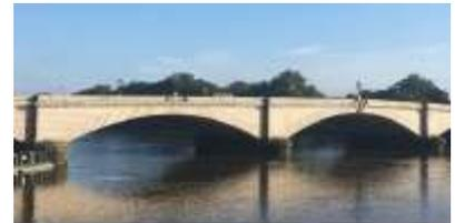
Look back at the Grade II listed **Putney Bridge (4)**. The present bridge, a five-span structure built of stone and Cornish granite, was designed by Sir Joseph Bazalgette and was opened in 1886. It was widened in 1933.
